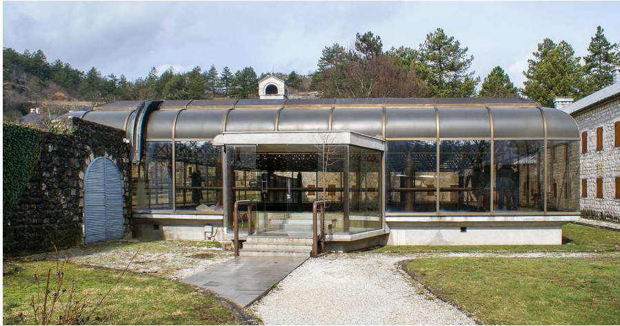
Fig. 16 The New, Current Pavilion of the Relief Map from the South (Mihailo St. Popović, 2020)
